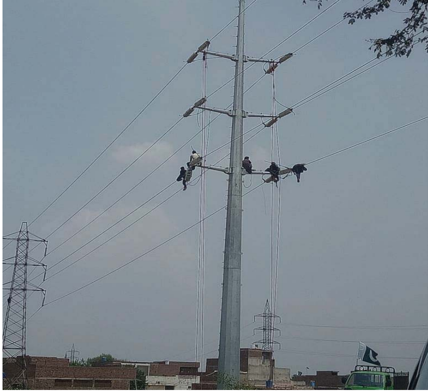
Work at 132KV Transmission Line in progress.
